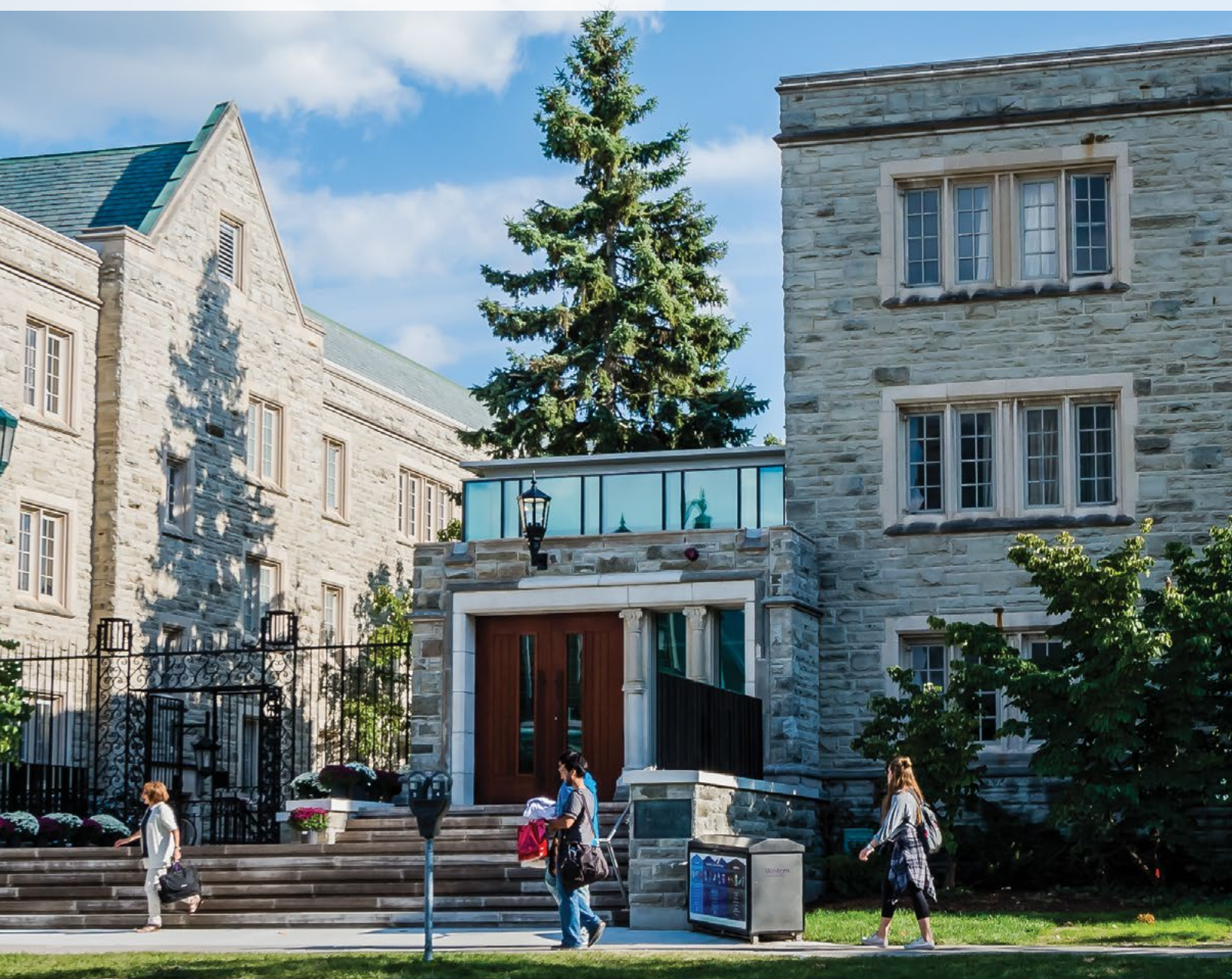
Medway-Sydenham Hall Residence
